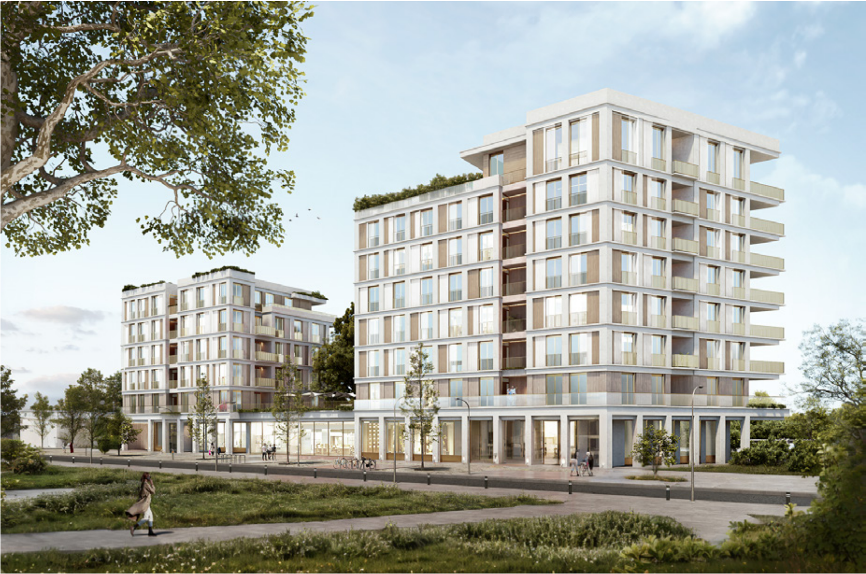
aprtment complex germany, 2024 bunni studio
