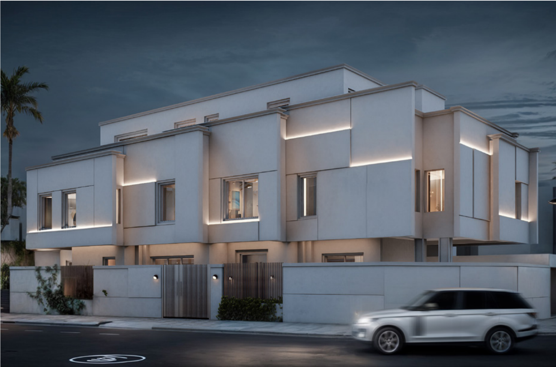
residential villa design jeddah, 2023 wadal w/ balkon works
